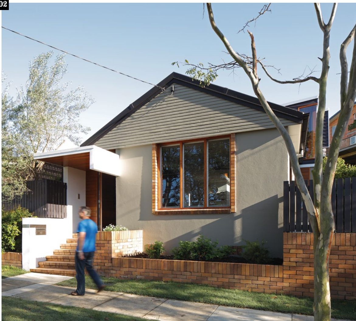
02 A relocated front door and additional entry structures enclose the southern courtyard.
