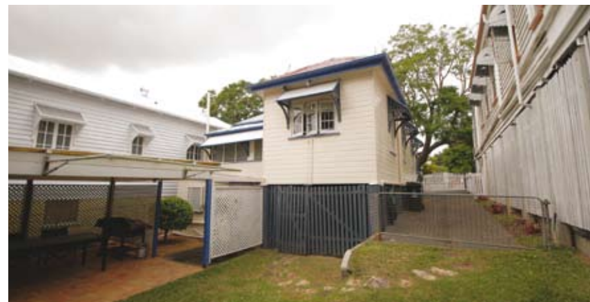
The rear of the Villiers Street residence prior to the extension. PHOTOGRAPHY ARKHEFIELD
